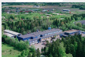
PEIRON OY STEEL FOUNDRY KOKEMÄKI, FINLAND
