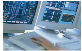
Process Control System
